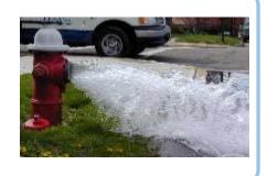
The field crew has scheduled the annual flushing of the water distribution system for **Monday**, **April 28 through Wednesday**, **April 30**. Annual flushing is a normal and required maintenance activity necessary to remove sedimentation and deposits in the water mains.
